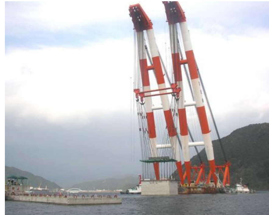
Caisson Installation Japan
